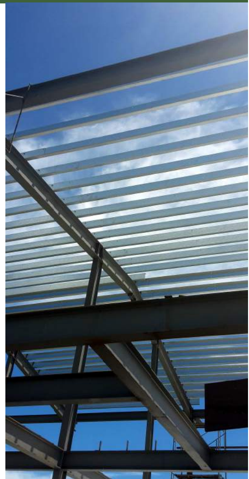
Training Room under construction in Tuvu
