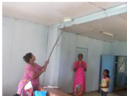
Painting the ceiling
