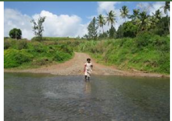
Mereani crosses the non existent “bridge”
